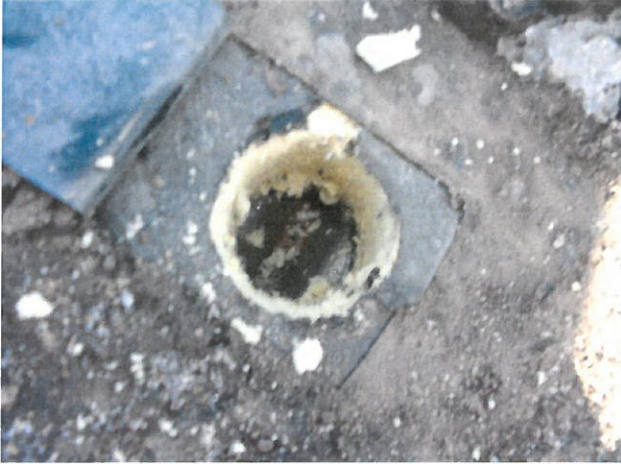
Roof Core Sample 039-01-Main Roof-NAD
