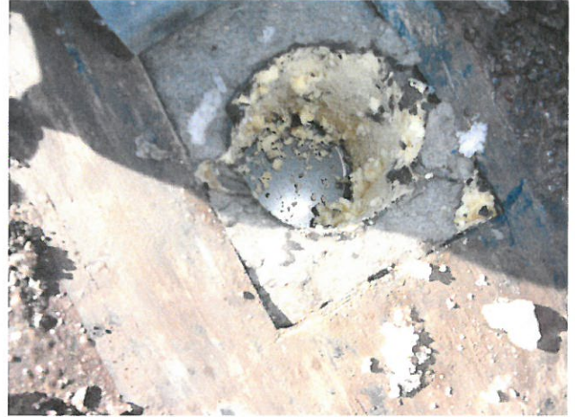
Roof Core Sample 039-02-Main Roof-NAD
