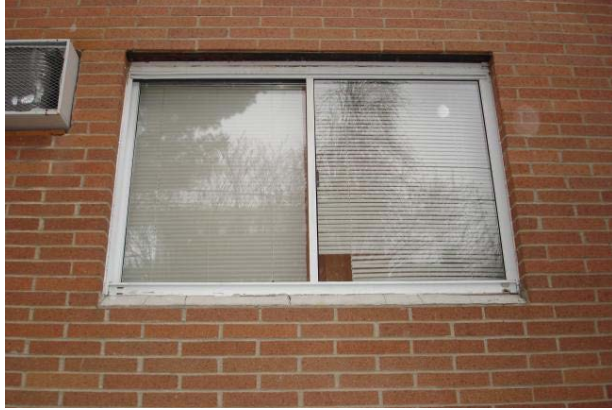
Photo 7 Missing precast window sill
