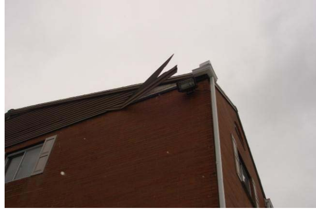
Photo 8 Damaged siding at roof gable
