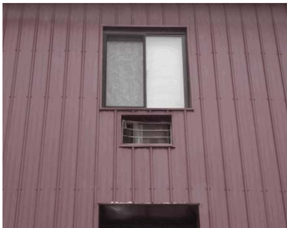
Photo 13 Thru-wall cooling unit- damaged
