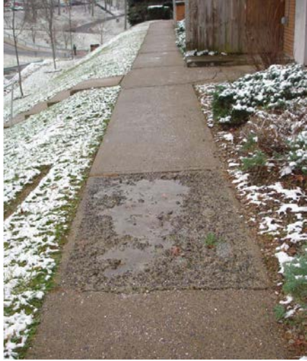
Photo 5 Concrete sidewalk spalling
