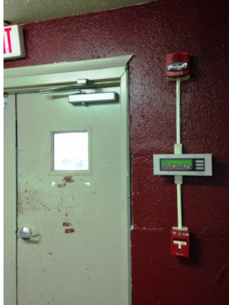
Photo 17- Fire alarm monitoring system
