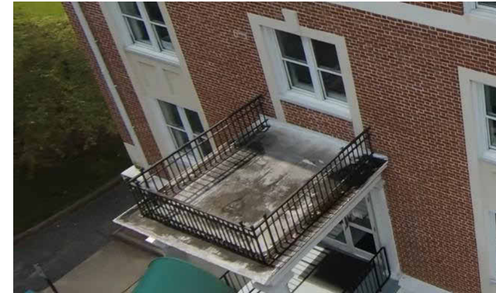
16 SIDE ROOF - EAST
