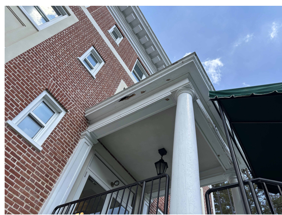
21 SIDE ROOF - WEST - SOFFIT
