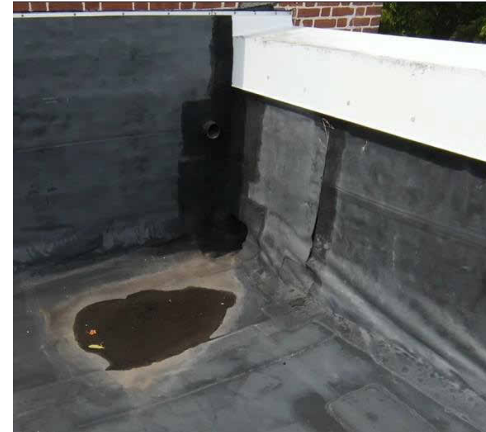
10 PARAPET WALL AND CAP
