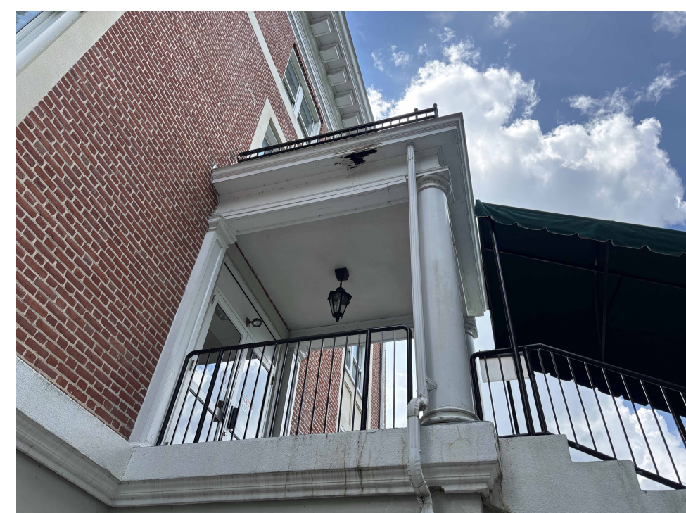
18 SIDE ROOF - EAST - SOFFIT
