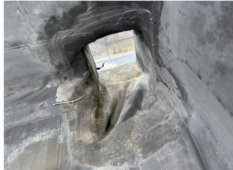
09 SCUPPER 1 (NW) INTERIOR
