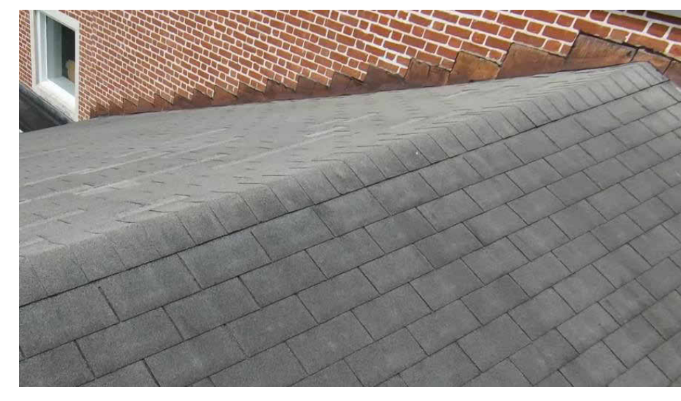
22 GABLE ROOF - STEP FLASHING SCALE: 1/2" = 1'-0" SHEET: AE-0.1
