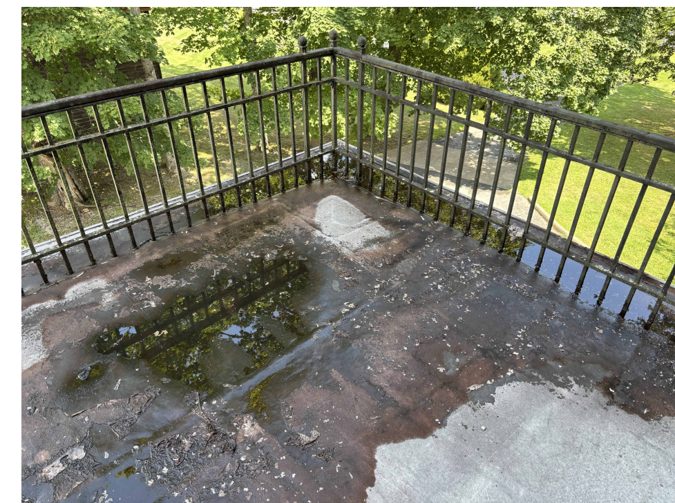
17 SIDE ROOF - EAST - RAILING
