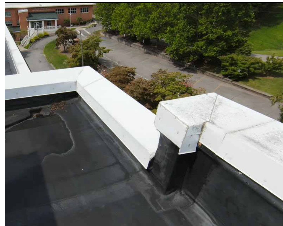
15 PENTHOUSE ROOF - PARAPET
