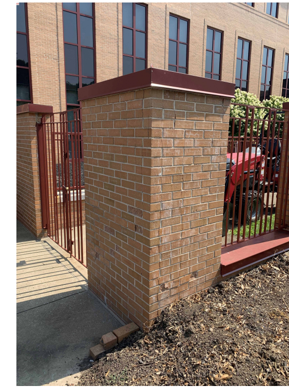
VIEW 23 - CLEAN AND REPOINT AREA AS NEEDED
