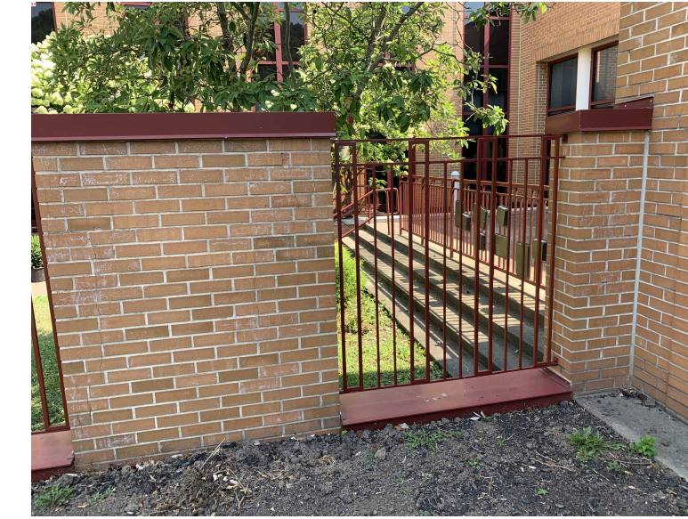
VIEW 27 - CLEAN AND REPOINT AREA AS NEEDED
