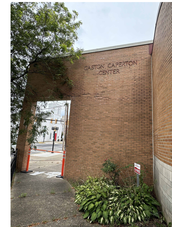
VIEW 16 - DEMOLISH PORTAL WALL - SEE A-4.1
