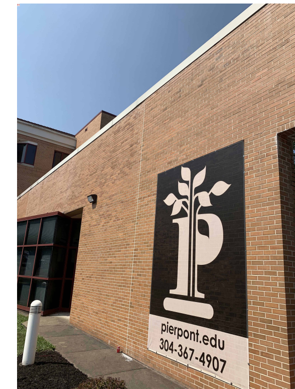
VIEW 17 - DEMOLISH PORTAL WALL - SEE A-4.1. SALVAGE SIGNAGE FOR OWNER
