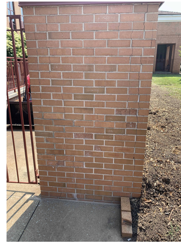
VIEW 22 - CLEAN AND REPOINT AREA AS NEEDED
