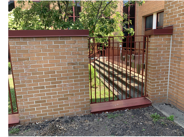
VIEW 27 - CLEAN AND REPOINT AREA AS NEEDED
